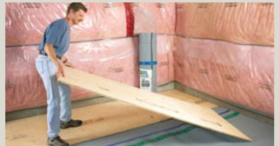
Laminate can be placed directly on DELTA®-FL.
